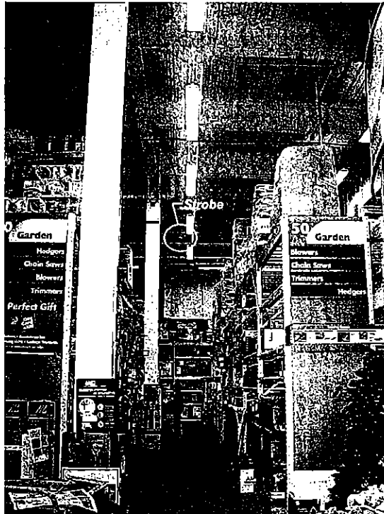
Photo 1 - Strobe Over Aisle (Reading, MA)
